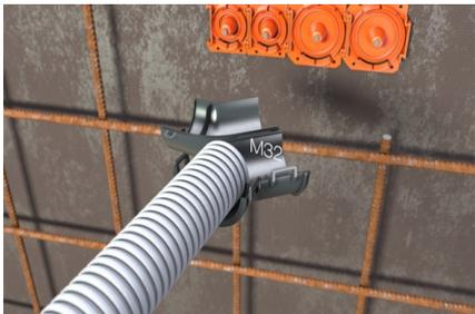
Open grommet (M20-M25) or elbow (M32-M40) and click in installation pipe.
