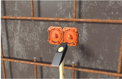
Wall mounting: Nail the front part to the formwork. Integrated nail fixation enables easy mounting.
