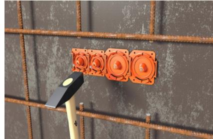
The front part can be firmly connected to other grommets and elbows by means of the plug-in system.
