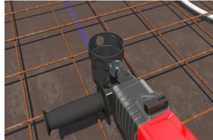
Open inserts for installation pipes
