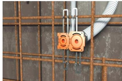
Front part enables firm and stable plug-in connection with other grommets or elbows.
